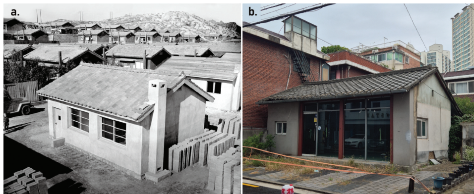
Figure 4. Typical urban-type National Housing units built by the UNKRA: (a) housing under construction by the UNKRA (December 1953); (b) remaining house in Jeongneung-dong (11 October 2024). Source: (a) UN Archives; (b) Authors.
