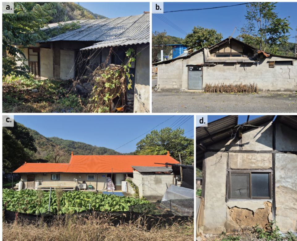
Figure 14. Remaining refugee houses in Yukdanri: (a) original structure preserved; (b) house expanded around the original building; (c) house extended along the length of the original structure; (d) original construction materials visible. Source: Authors.
